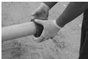
Stab mold onto pipe
