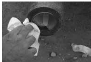
Clean excess paste from mold
