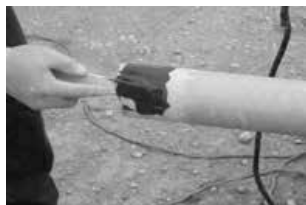
Apply paste to pipe
